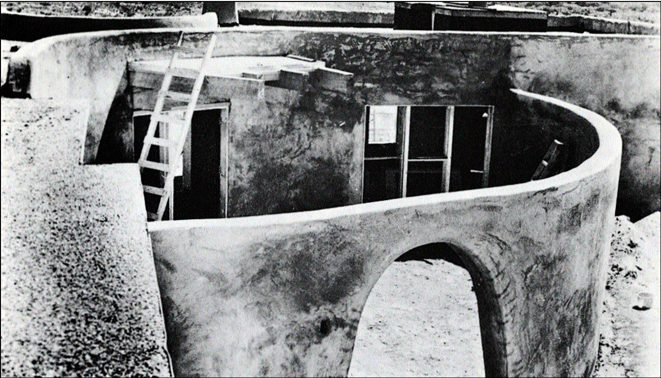
House under construction in Albuquerque, New Mexico.
